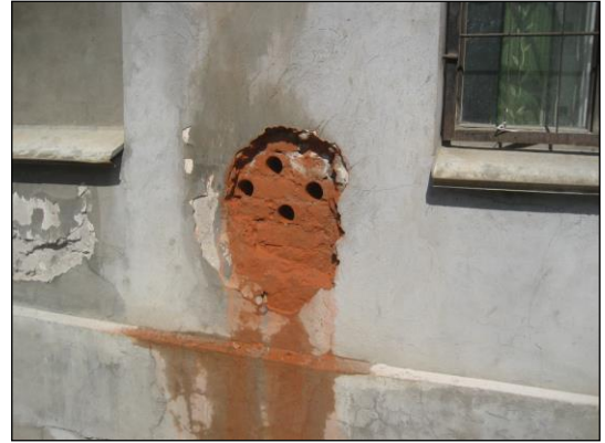
Figure 5. Sampling sites from building walls to the address: Zhukova street 17
